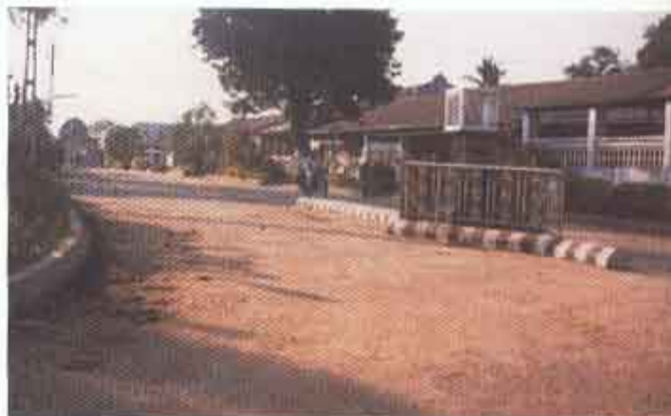
Raghuvirbhai Kevadbhai Bhagat Compound Wall, Kelvekuva
