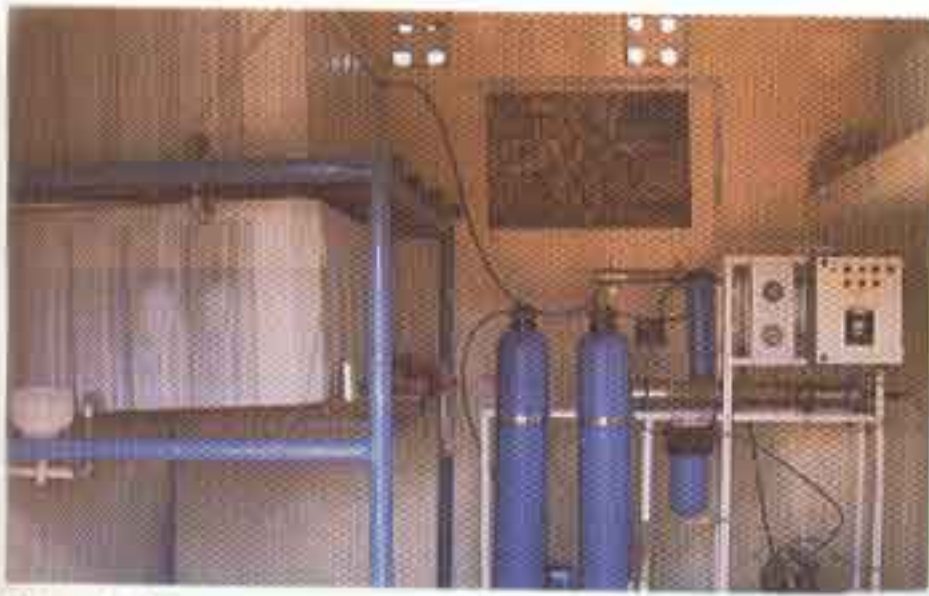
Mahopatsinh Narpatsinh Vashi Filter Plant, Raiyma, Rs. 0.50 lac
